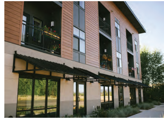
Driggs' Depot Square, completed in 2023, includes thirty deed-restricted affordable apartments, as well as retail and business incubator spaces.
